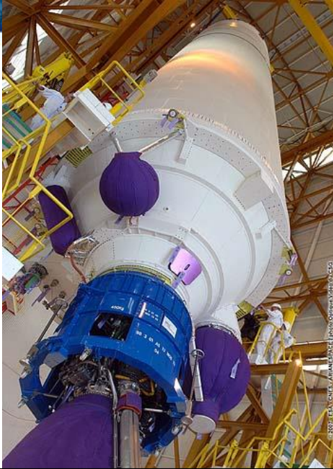
Kourou: hoisting the EPC in the Launcher Integration Building (BIL) © ESA/ARIANESPACE/Service optique CSG
